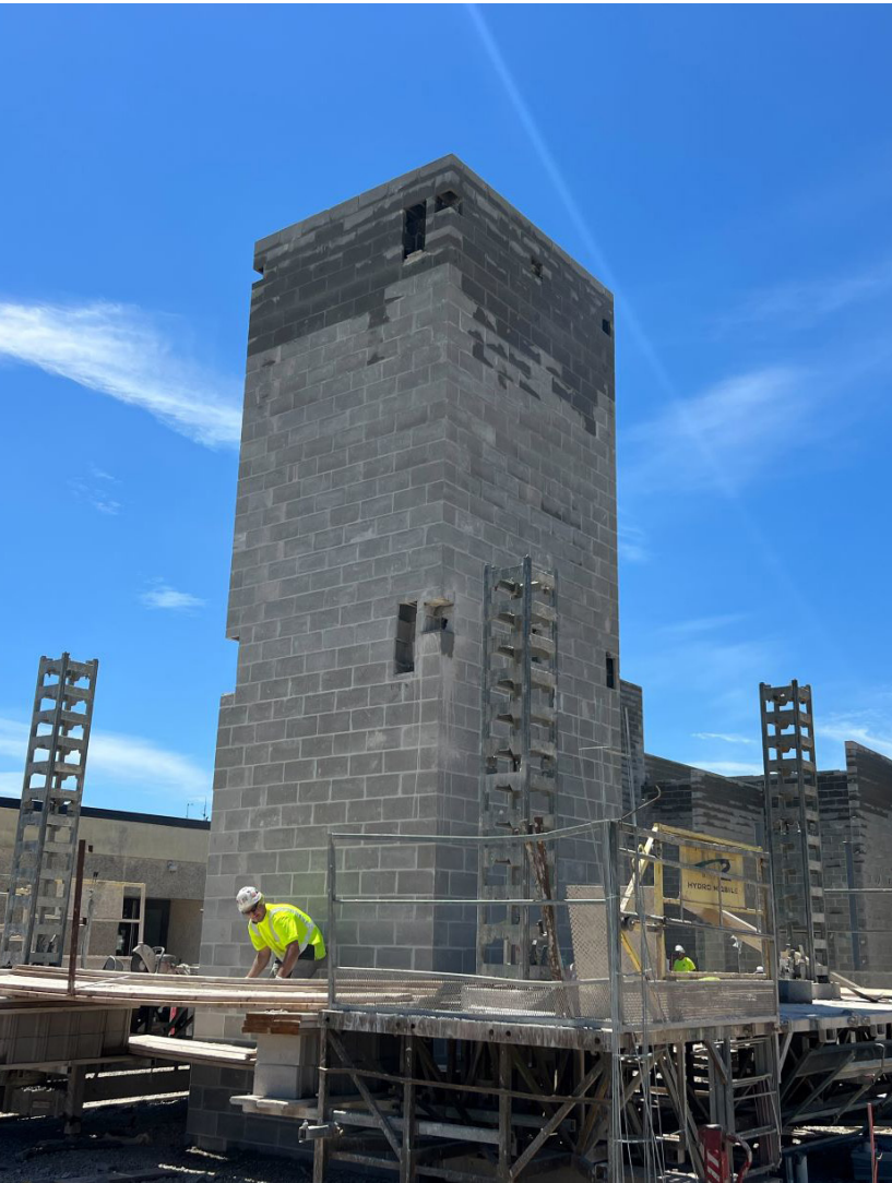
MASONRY ELEVATOR SHAFT COMPLETE
