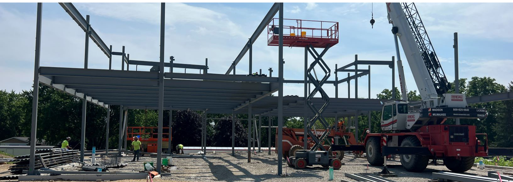
UNIT F STEEL ERECTION IN PROGRESS
