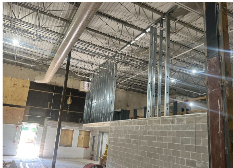
MEZZANINE WALL FRAMING IN PROGRESS
